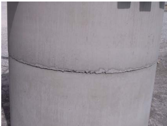
Carefully lower sections together (May or may not see "squeeze out")
