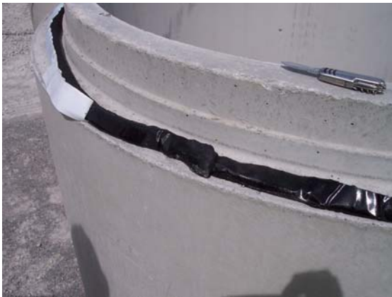
Place sealant on MH section & remove plastic Knead ends together to form a continuous strand Do not overlap (Cut sealant to length in needed)
